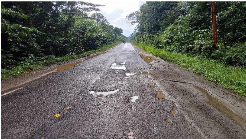
Gambar 1. Lubang (Potholes)
